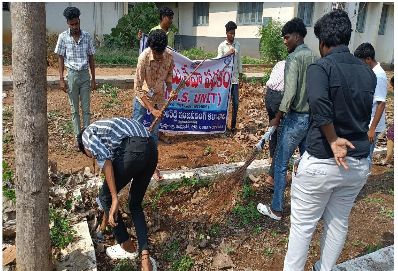
LBRCE NSS Volunteers clean the potholes
